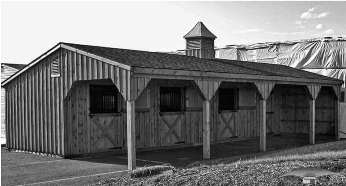
SHED ROOF WITH 8 FOOT ROOF EXTENSION
