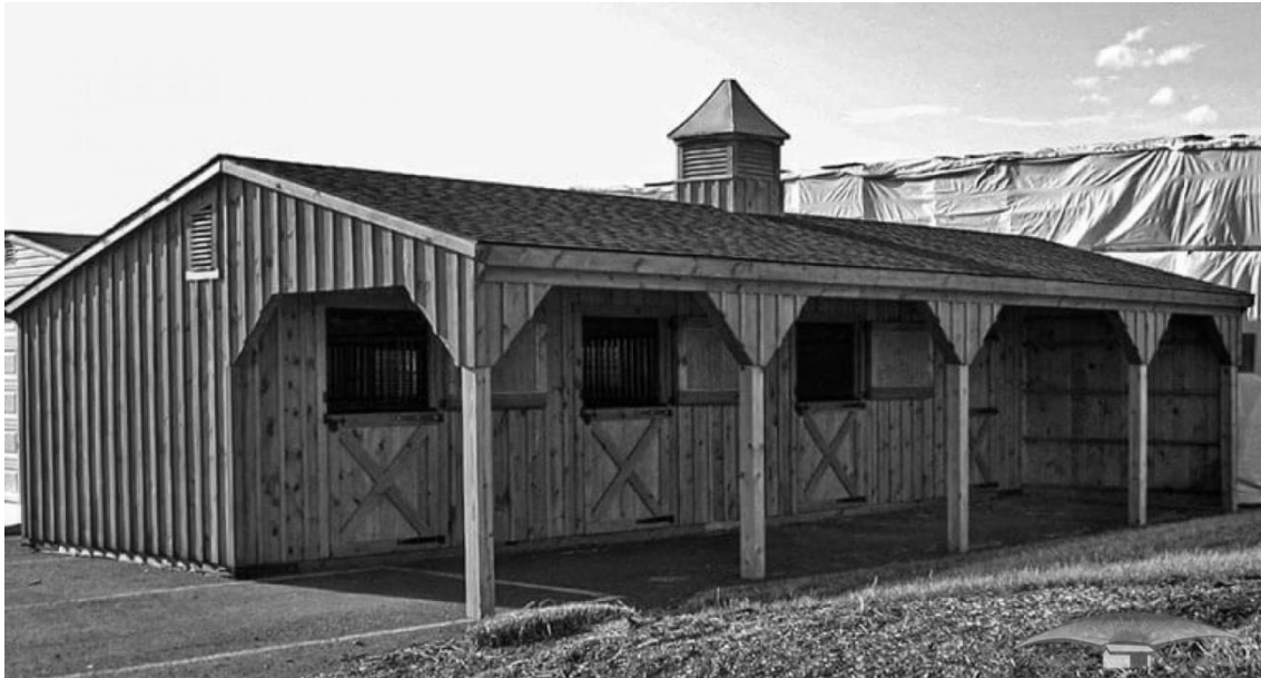
SHED ROW WITH 8 FOOT ROOF EXTENSION
