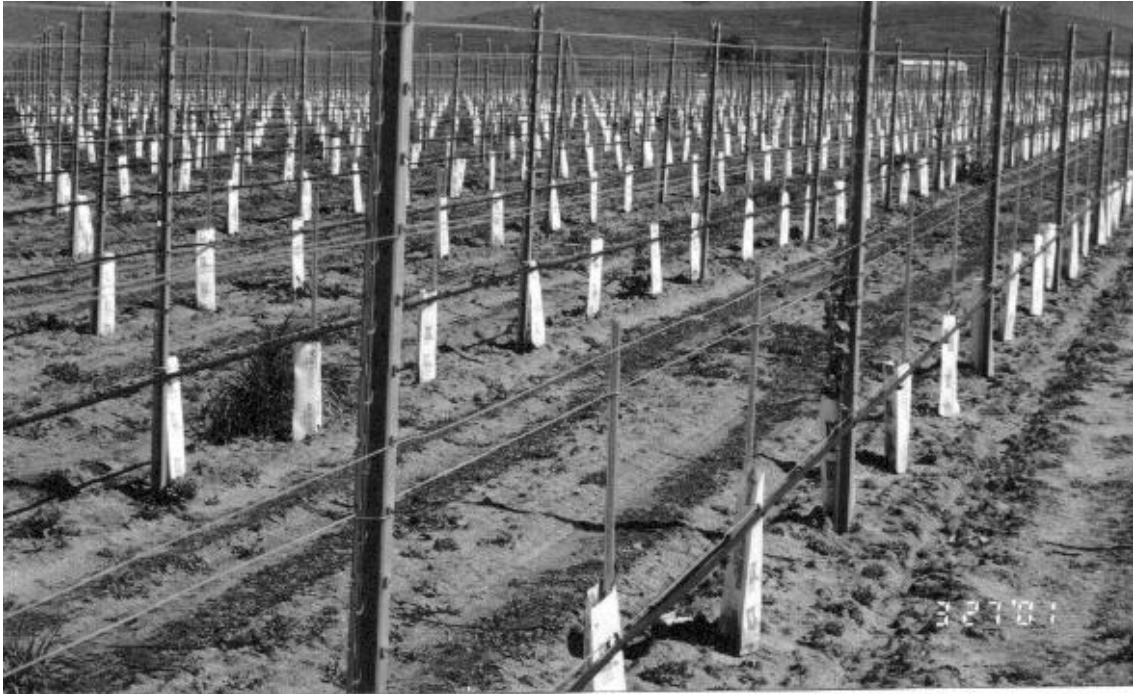
8' vertical line post with 4' T-posts in between
