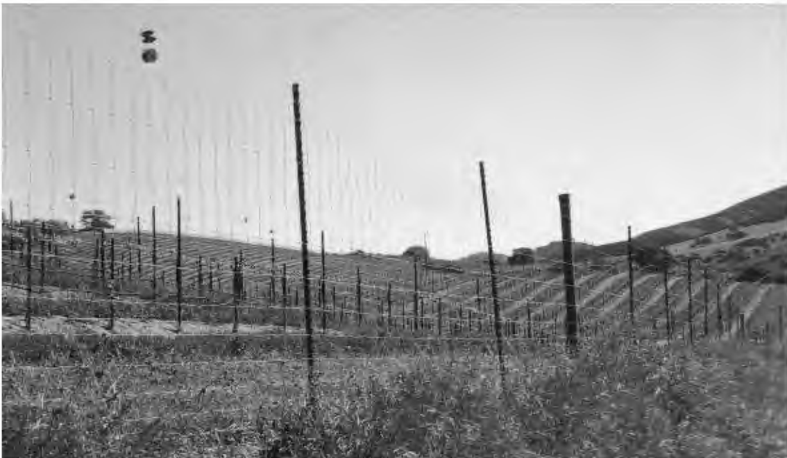
7' Deer fence made with 9' T-post and 9' wood stakes 6 ½' woven wire with 2 barbed wires on top and steel gates at drives
