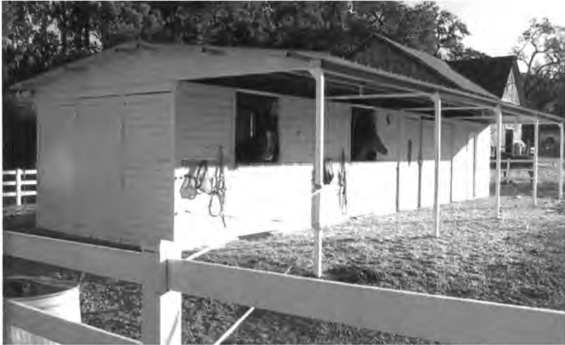
SHED ROW WITH 8 FOOT ROOF EXTENSION
