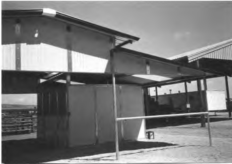
GABLE ROOF—RAISED BREEZEWAY WITH ROOF EXTENSION
