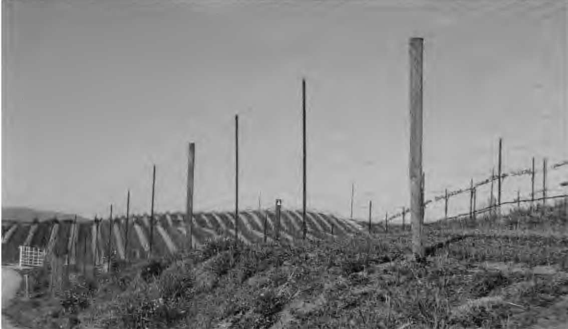
7' Deer fence made with 9' T-post and 9' wood stakes 6 ½' woven wire with 2 barbed wires on top and steel gates at drives
